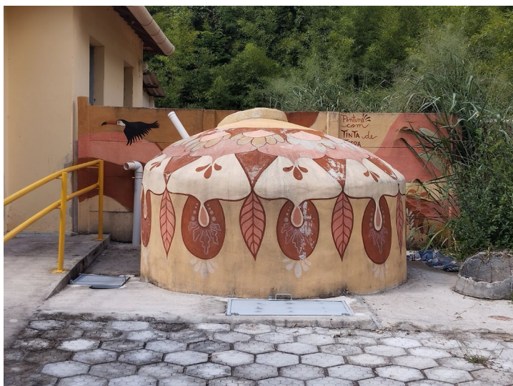
Rainwater collection cistern painted with natural dyes
